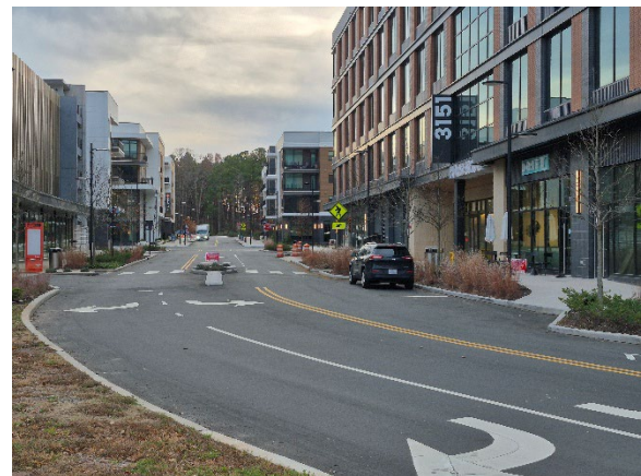
Development underway at HUB RTP
